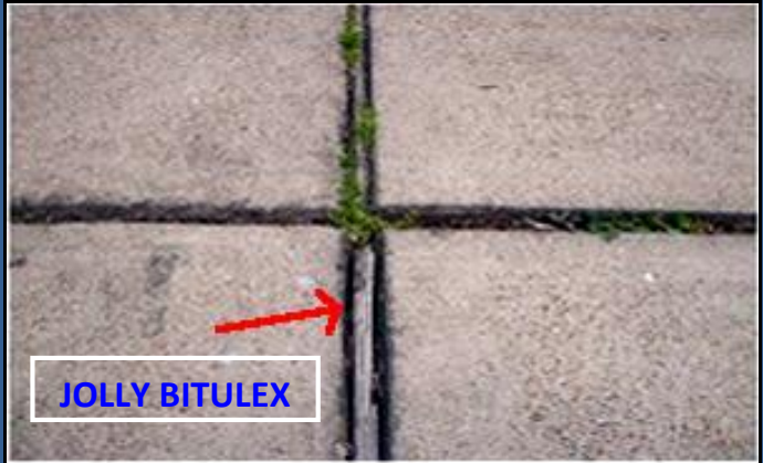
JOLLY EXPANSION JOINT FILLER IN SIDE WALK
