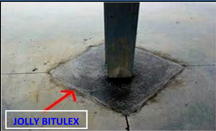
JOLLY EXPANSION JOINT FILLER IN COLUMN JOINTS
